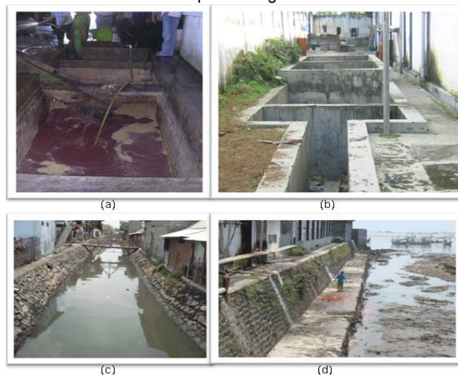
Fig. 1. Pictures showing wastewater facility at the source (a, b), open ditch carrying wastewater (c) and final disposal into the sea (d)
